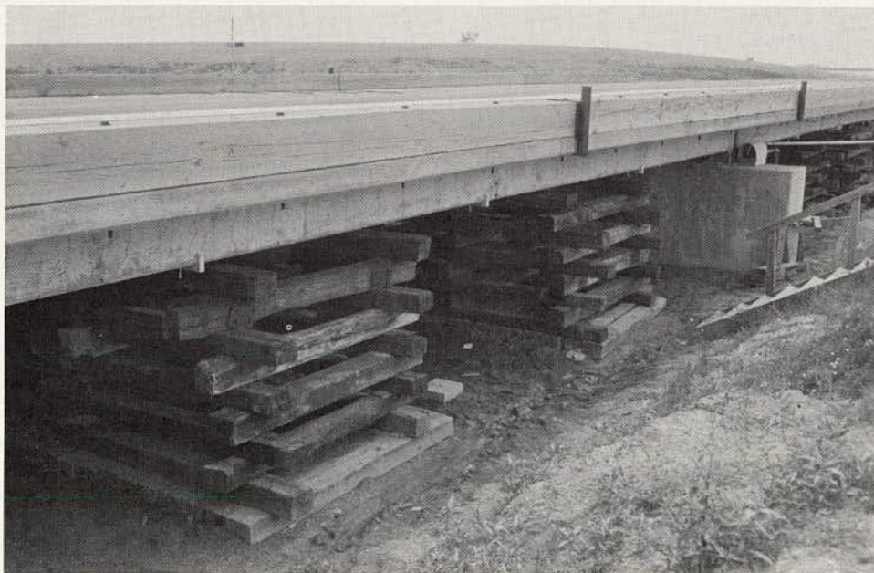
Figure 56. Safety cribs under Bridge 7B.
