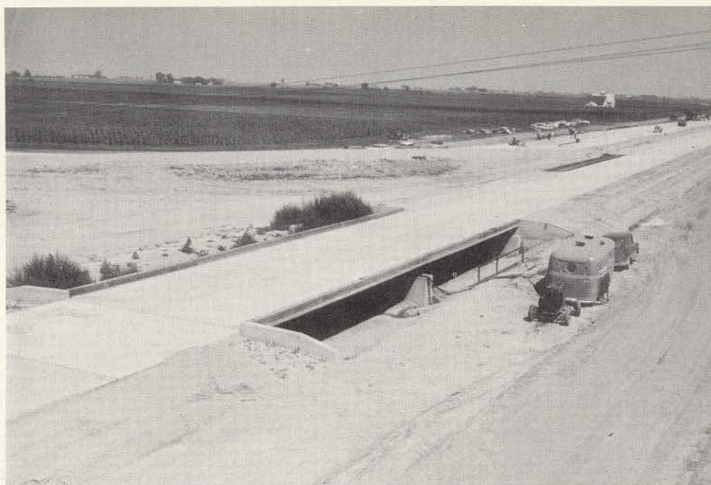
Figure 10. Set of four completed bridges.
