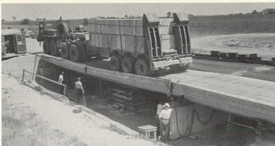
Figure 60. Special vehicle with extra heavy load during test to failure with increasing loads.
