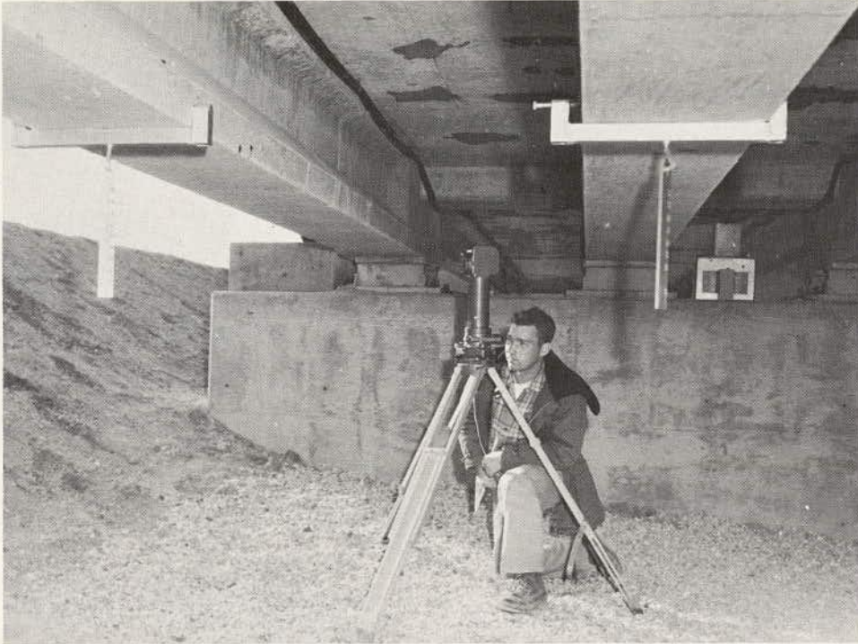
Figure 19. Brackets and scales for measurement of beam elevations.
