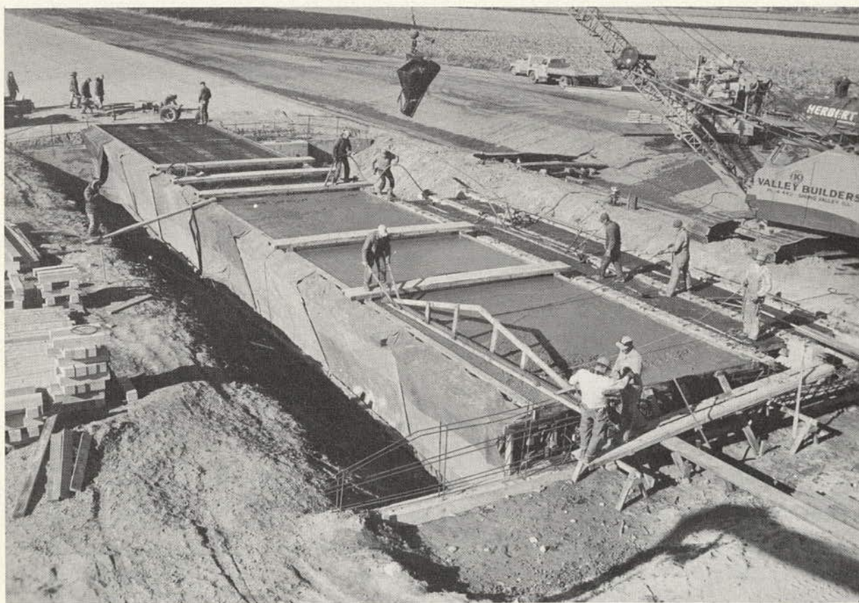
Figure 11. Casting a concrete slab.
