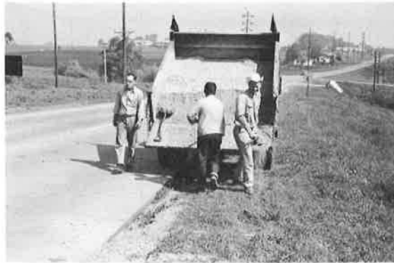
Figure 24. Spreading aggregate in edgerut by hand.
