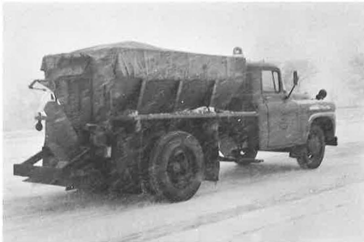
Figure 38. Truck with spreader bed salting roadway surface.
