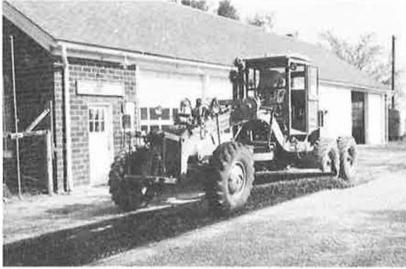
Figure 10. Motorgrader mixing aggregate and asphalt.
