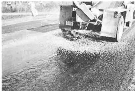
Figure 22. Truck with spreader bed applying aggregate.
