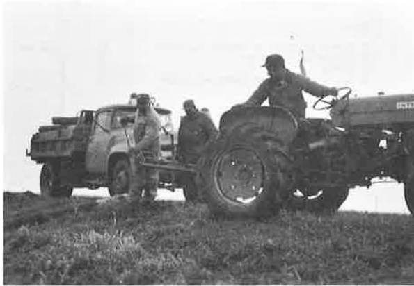
Figure 41. Tractor with power auger digging hole for guidepost.
