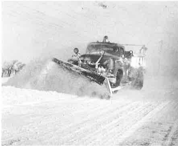
Figure 32. Light duty truck with one-way plow plowing shoulder.
