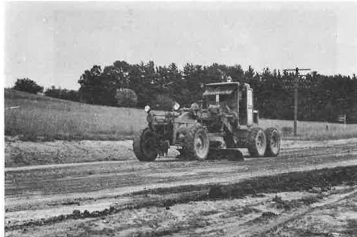
Figure 16. Motorgrader blading gravel surface.
