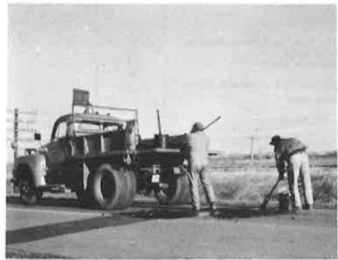
Figure 13. Priming hole and spreading cold mix by hand.
