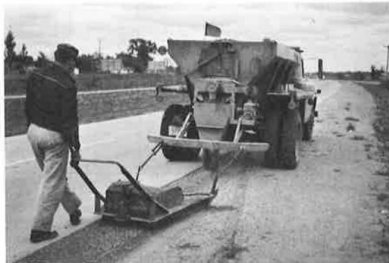
Figure 25. Spreading aggregate in edgerut with drag.
