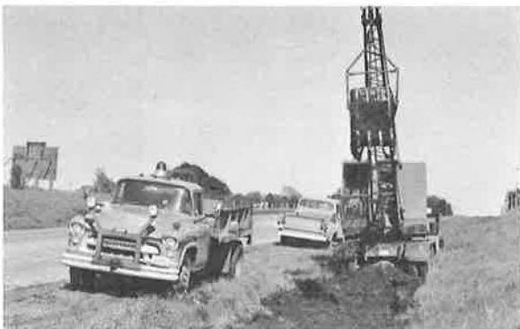
Figure 28. Dragline cleaning sod and soil from ditch.
