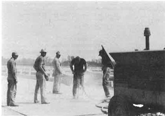
Figure 17. Drilling hole with jackhammer.
