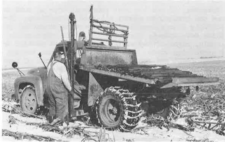
Figure 35. Driving snow fence post with power driver.
