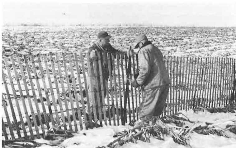
Figure 36. Erecting snow fence.
