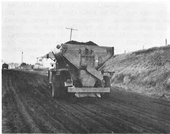
Figure 11. Truck with spreader bed spreading aggregate in ruts.
