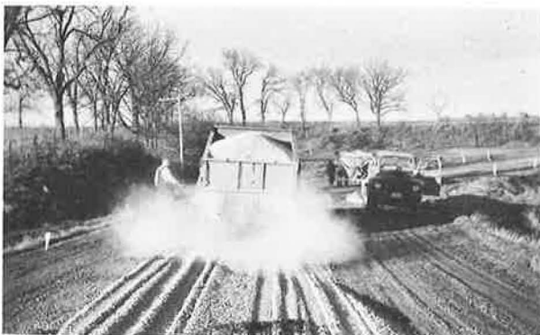
Figure 20. Truck spreading aggregate.
