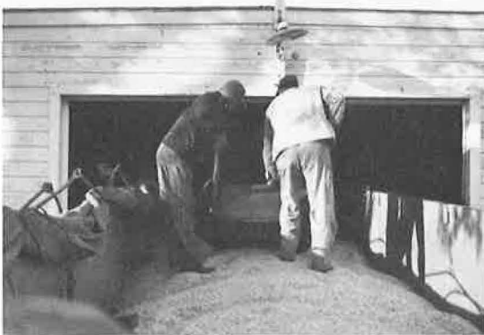
Figure 9. Unloading salt with drag bucket.
