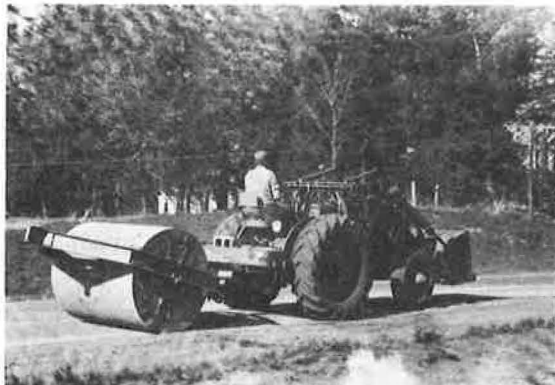
Figure 23. Tractor and steel wheel roller rolling sealed area.
