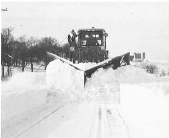
Figure 33. Motorgrader with Vee plow plowing drift on roadway surface.
