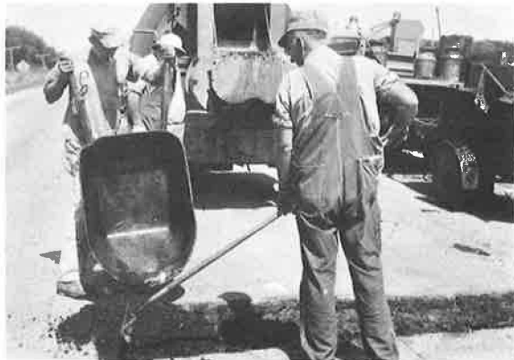
Figure 14. Hand spreading bituminous hot mix.
