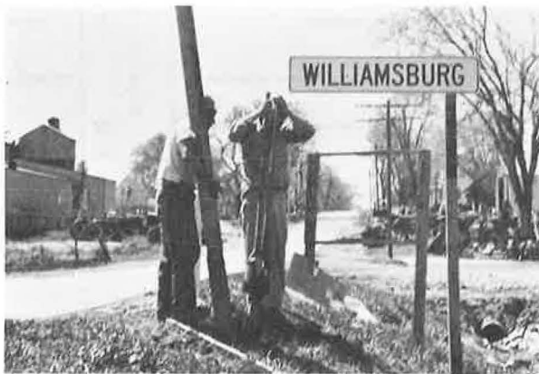
Figure 42. Digging hole for sign post by hand.
