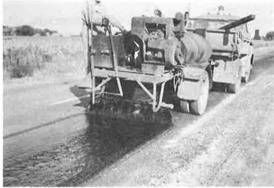
Figure 21. Distributor spraying asphalt.
