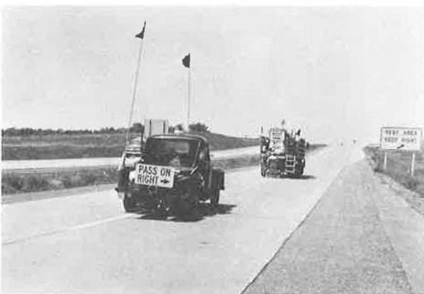
Figure 40. Paint truck and pickup truck used for placing warning blocks.
