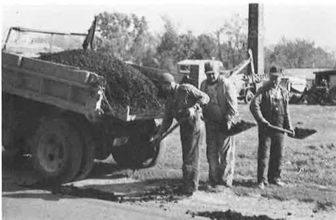
Figure 27. Spreading cold mix in edgerut by hand.
