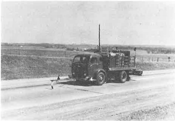
Figure 39. Paint truck putting down centerlines.
