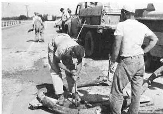
Figure 18. "Priming" hole before starting to pump mud.
