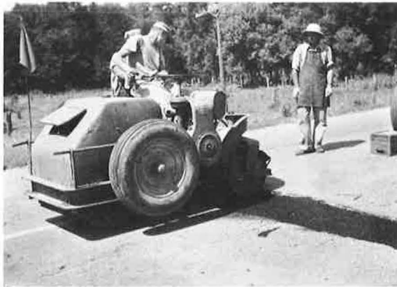
Figure 15. Self-propelled roller compacting hot mix patch.
