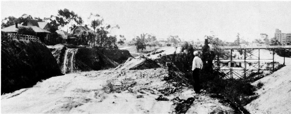
Figure 10. Sears interchange, before.
