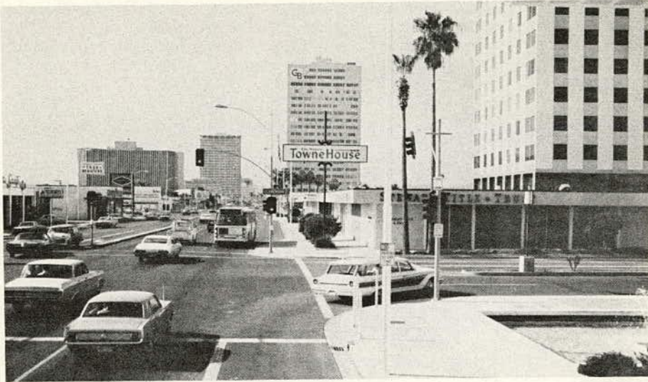
Figure 1. Recessed bus bay, Phoenix, Ariz.
