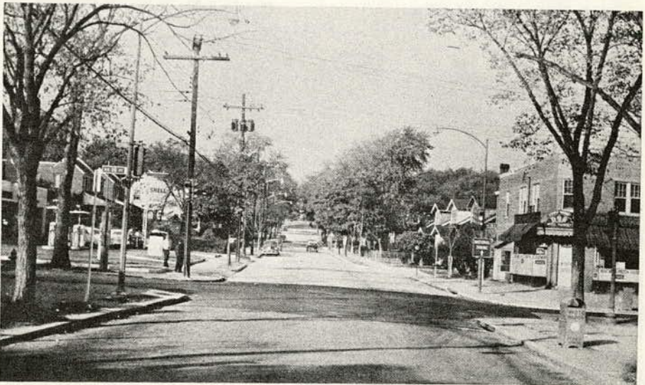
Figure 7. After bus bay construction.
