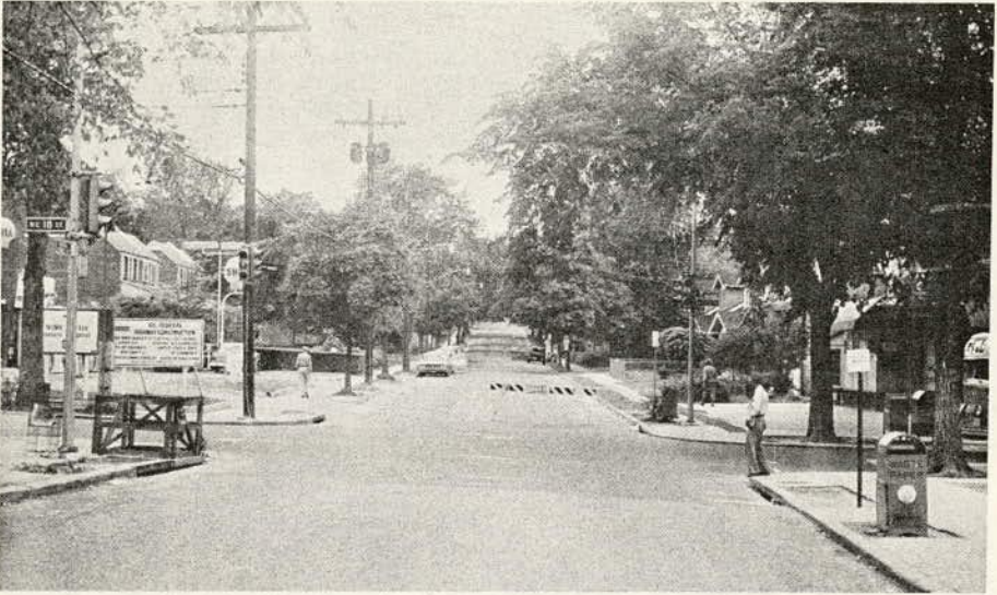
Figure 6. Before bus bay construction.
