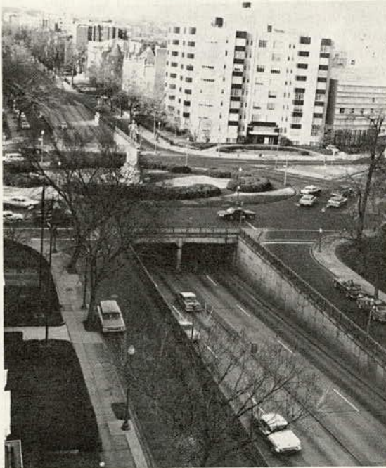
Figure 4. Example of a traffic circle underpass, 16th and M Streets, N.W., Washington, D.C.
