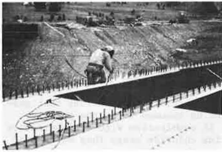
Figure 2. Typical form support and sheet metal screw connection, used in push-out tests conducted by Barnott and Jones (4).
