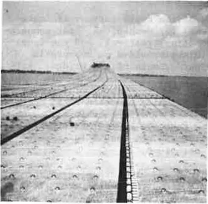
Figure 1. Prestressed panel subdecks in place on a bridge deck in Texas.
