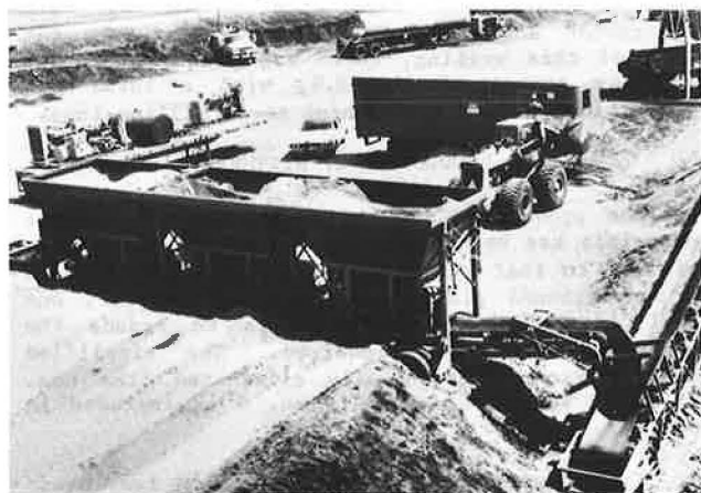
Figure 13. Three-bin feeder system also part of new Shearer plant system
