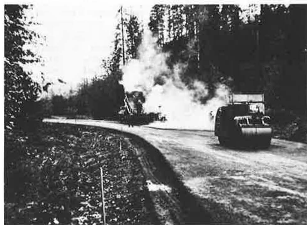
Figure 16. Paving operation in progress in Washington State at 16 F.
