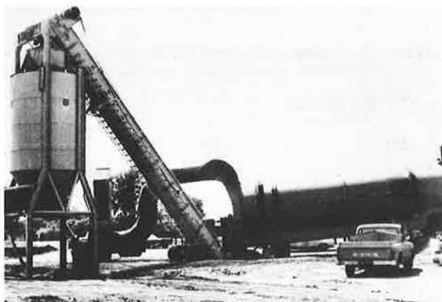
Figure 14. Slat conveyor, surge silo, and dryer-drum components of Shearer plants
