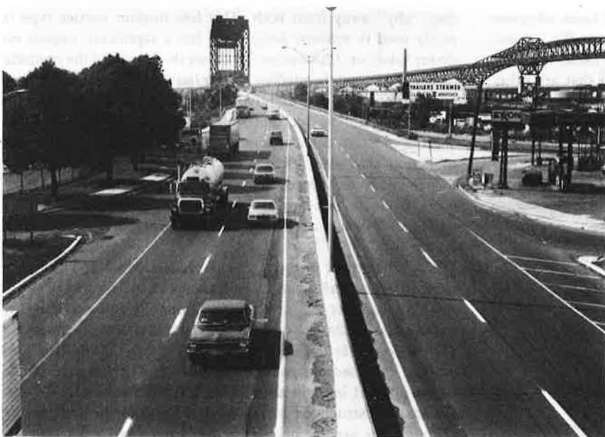
Illustration 3-11. This cross section illustrates ideal conditions of lane width and lateral clearance. The concrete median barrier does not cause vehicles to shift their lane position, and therefore would not be considered an "obstruction."
