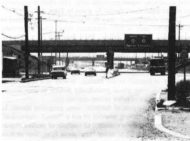
Illustration 7-5. Note the bridge pier located in the center of a normally undivided suburban multilane highway. Vehicles will tend to adjust their position in adjacent travel lanes to avoid traveling too closely to the abutment.
