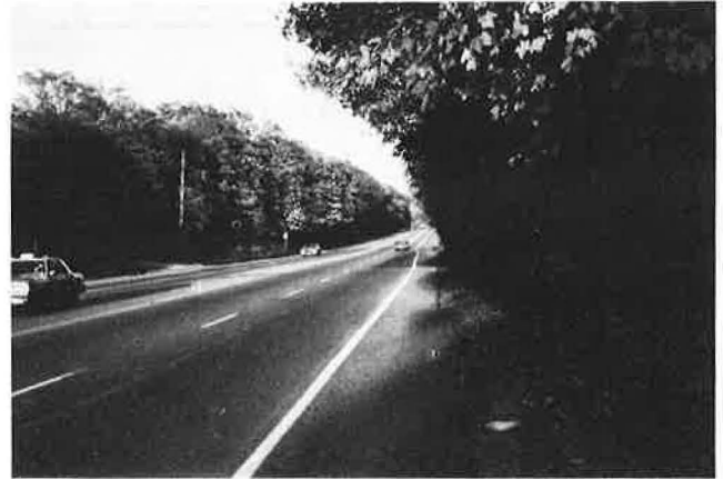
Illustration 7-8. This undivided multilane highway has no obstructions at the roadside closer than 6ft to the travel lanes. The impact of opposing flow on median lanes is not a "lateral obstruction," and is accounted for elsewhere in the procedure.
