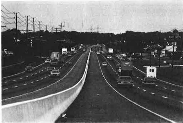
Illustration 7-7. This divided multilane highway displays "ideal" geometric conditions, with no median or roadside obstructions to influence flow.
