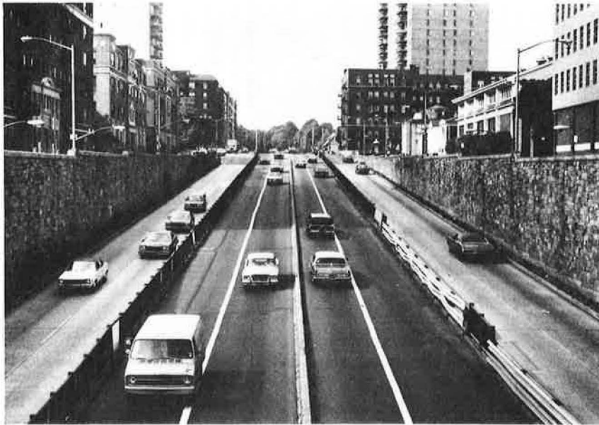
Illustration 3-1. Vehicles shy away from both roadside and median barriers, driving as close to the lane marking as possible. The existence of narrow lanes compounds the problem, making it difficult for two vehicles to travel alongside each other.
