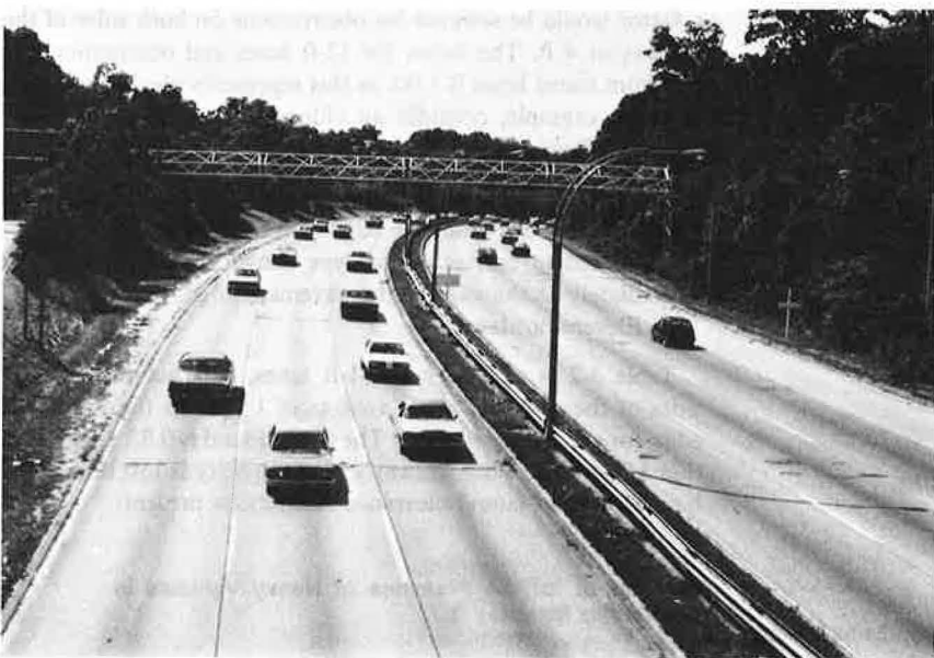
Illustration 3-12. The freeway section shown here is also ideal with respect to lane width and lateral clearances. The W-beam median barrier is another type of barrier which generally does not cause vehicles to shift their lateral lane placement, and also would not be considered an "obstruction" in most cases.
