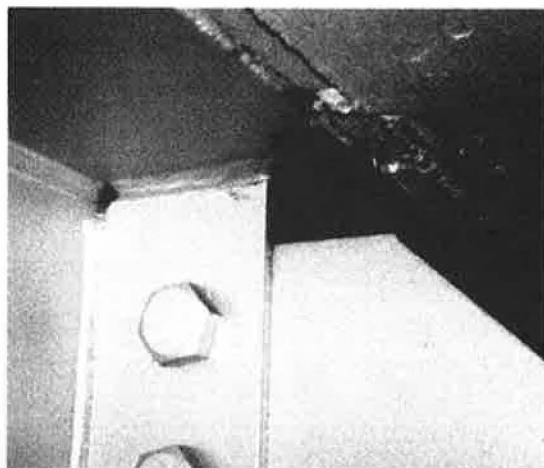
Figure 3: Cracked connection weld between girder top flange and diaphragm connection stiffener.
