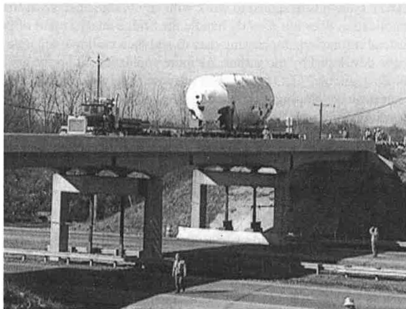
Figure 3: Temporary substructure supports.
