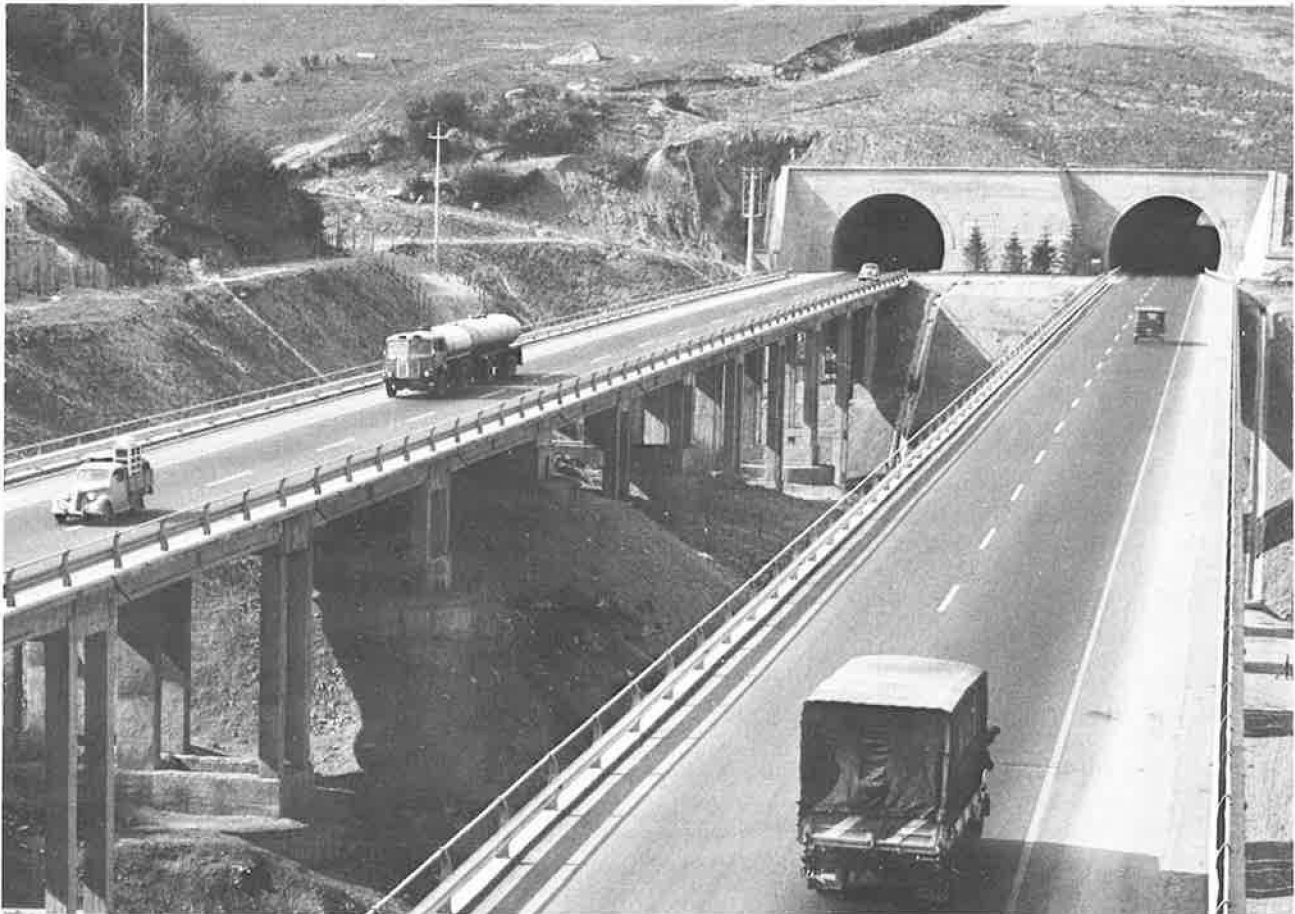
Elevated structure and tunnels on the autostrada between Bologna and Florence, Italy.
