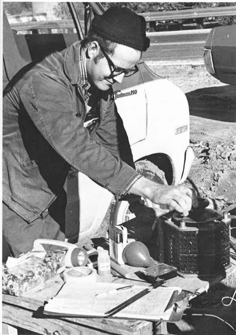
Will Gilliland operates the transformer used to regulate electrical current in bridge deck for removing chloride.
