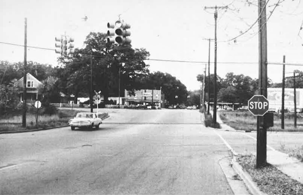
Examples of traffic control devices that do not conform to the Manual on Uniform Traffic Control Devices are (a) stop sign used in conjunction with traffic signal, (b) single signal face for approaching traffic, (c) inadequate vertical clearance of signal head, (d) no railroad cross buck for approaching traffic, and (e) poorly maintained pavement markings and no advance markings for the railroad crossing.
