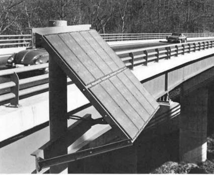
1 Facing south for the maximum exposure to sunlight, the collector has a design output of 33 amperes.
