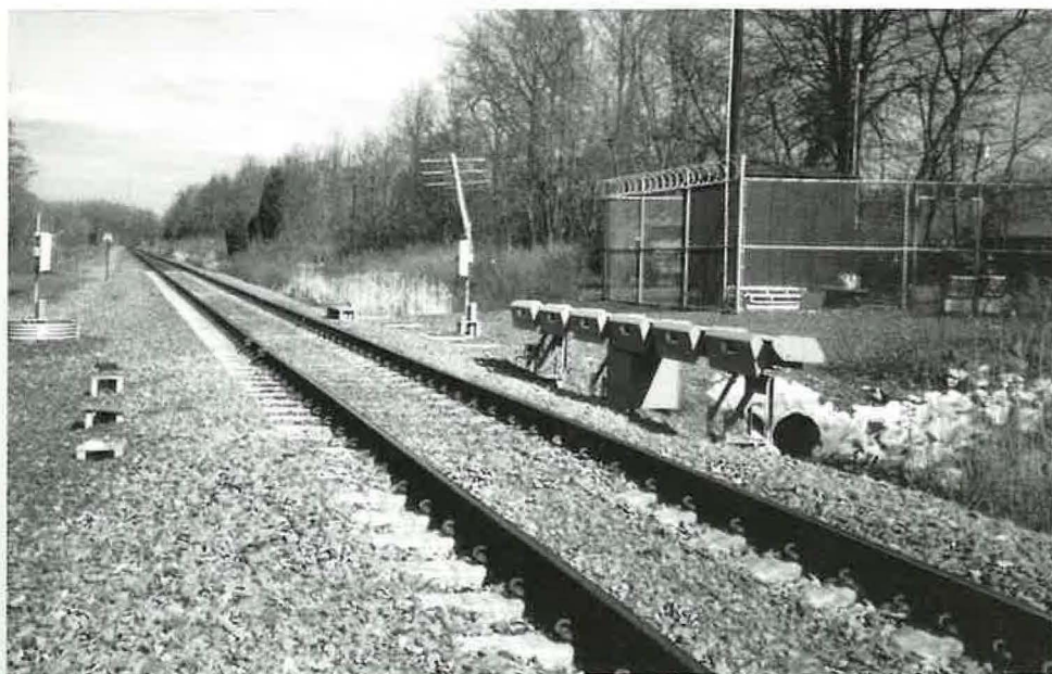
FIGURE 4 Development and implementation of new-generation wayside acoustic bearing-defect detectors are expected to facilitate early detection of defective bearings.
