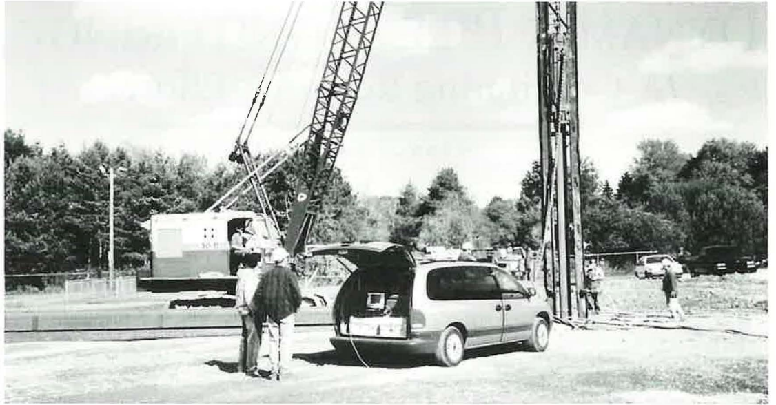
FIGURE 1 Dynamic pile monitoring with pile driving analyzer at job site, Cleveland, Ohio.
