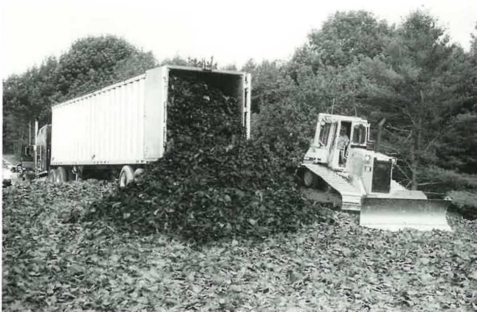
FIGURE 1 Spreading tire shreds for Portland Jetport Interchange in Maine using a small bulldozer.
