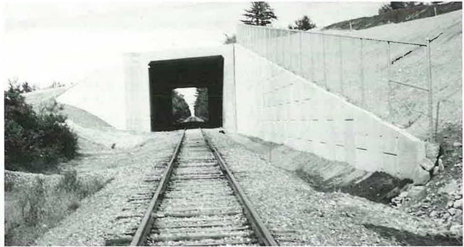
FIGURE 2 Completed rigid-frame bridge on Route 196, Topsham, Maine.
