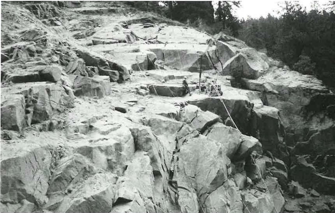
On-slope stabilization of an unstable rock slope using a bench drill to install rock bolts and dowels in north central Washington State.
