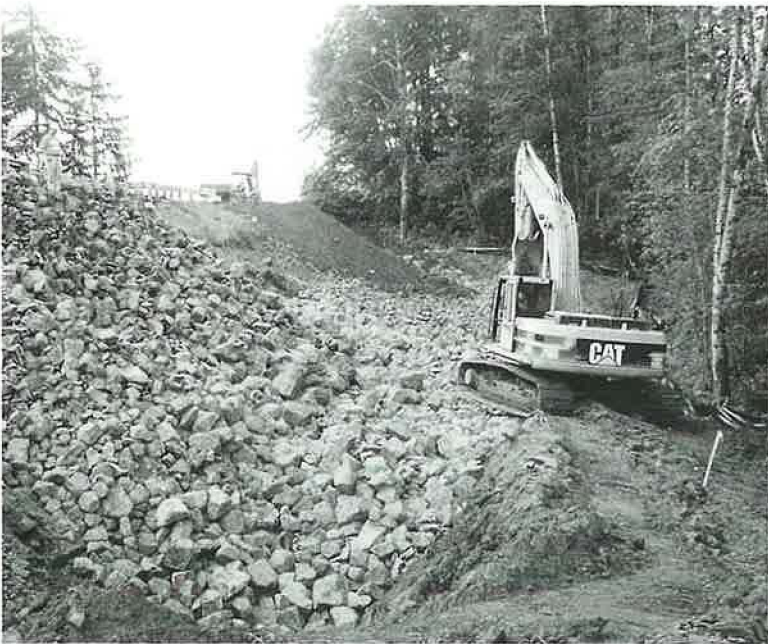
Construction of a rock shear key to stabilize an embankment affected by a landslide in southwest Washington State.
