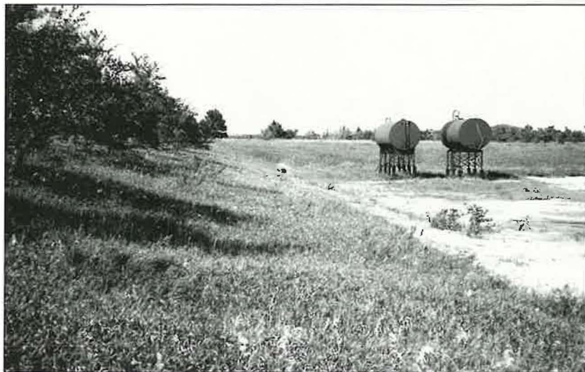
FIGURE 1 Earthen berms around an entire storage yard can contain spillage from road oil tanks. Smaller berms can surround the immediate loading area and the tanks.
