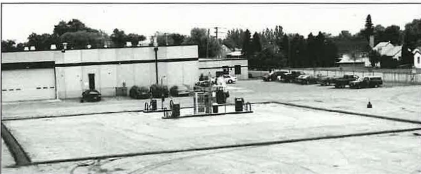
FIGURE 2 Low-lying bituminous berms in loading area for diesel and gasohol underground storage tanks can control spills but allow easy passage of vehicles. A blockable drain at low point of berm empties runoff from precipitation.
