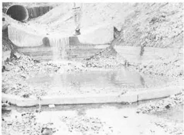
Figure 1. Assembled modular energy dissipator.
