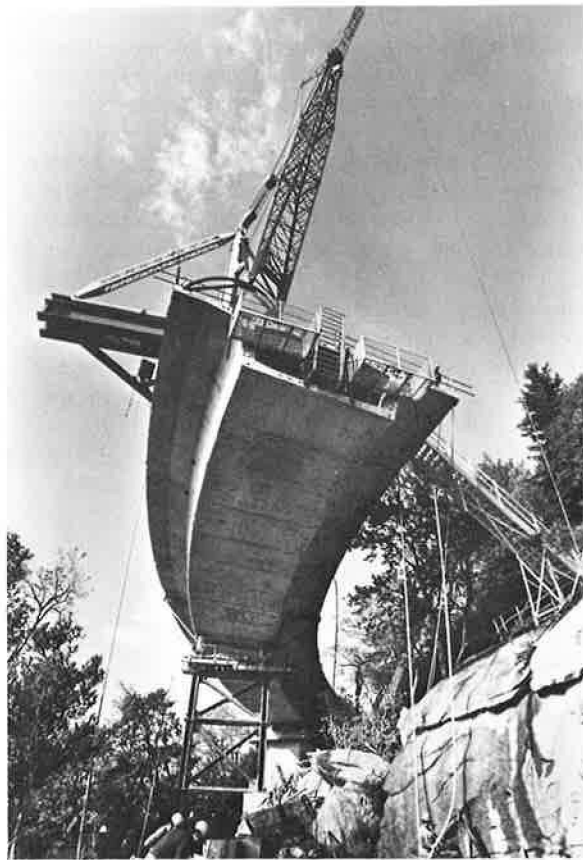
The bridge turns on a 250-ft radius around a rock outcrop. A stiffleg derrick is at the lead of the cantilever with a steel temporary support shown in the background.
