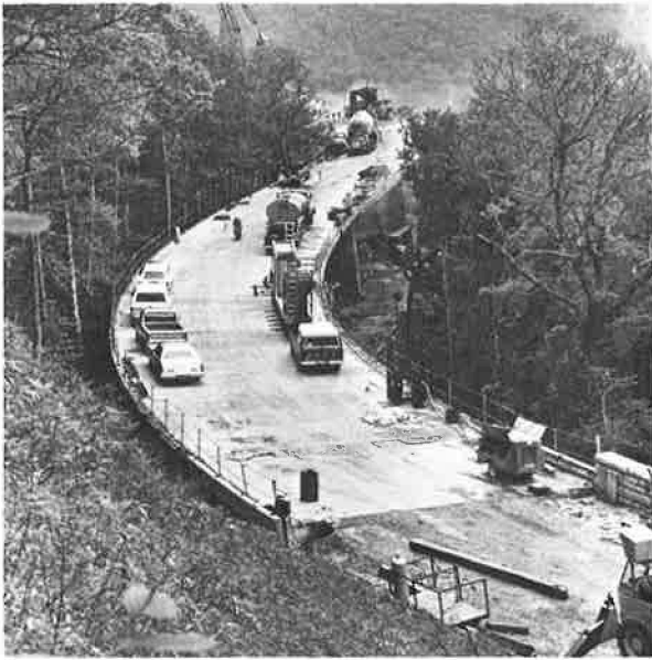
Bridge construction is shown as it reaches the halfway point. Exact geometry and casting controls enabled the structure to be erected in virtual conformance with the theoretical geometry.
