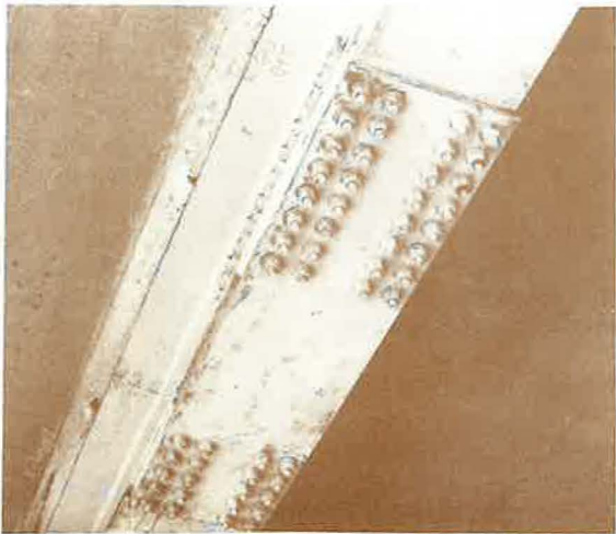
8. Bolted splice used to repair beams with severe fatigue cracking. This method was used to repair several cracked beams at a cost of approximately $2000 each, in the Yellow Mill Pond Bridge.
