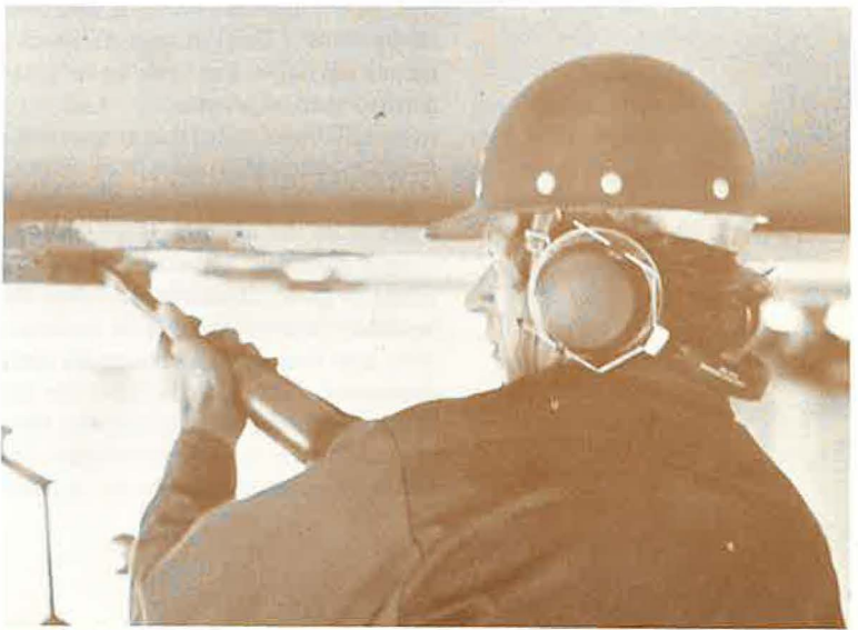
9. Research at Lehigh University has shown that air-hammer peening along the weld toe at the end of a cover plate can extend significantly the fatigue life of a bridge beam. At a cost of about $50/joint, peening was used to retrofit some 700 cover plate ends in the Yellow Mill Pond Bridge, thus avoiding almost certain fatigue cracking problems and the need for costly bolted splices in this heavily traveled structure.
