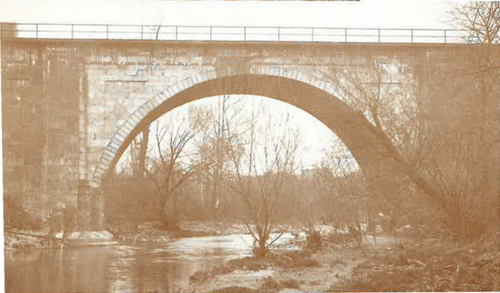
4. Stone arch bridge (Carrollton Viaduct) carries the original main line of the B&O Railroad over Gwynn's Falls. This is the first railroad bridge built in the United States, 1829. (Courtesy of B&O Railroad Museum Archives)
