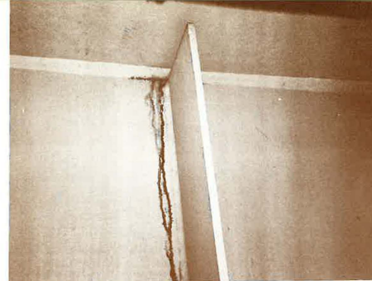
13. Cracking can be seen in this photograph along the flange-web weld near the top of the transverse stiffener, with rust stains running down the web. A retrofit technique developed by John Fisher of Lehigh University has been used to arrest the growth of fatigue cracks and to reduce the severity of out-of-plane deformations in many bridges. This technique involves drilling holes at the ends of the crack and increasing the gap between the flange and the end of the transverse attachment. The total cost of applying this retrofit technique to fatigue-prone members in 36 bridges in Iowa was estimated to be less than the cost of the removal and replacement that would have been required if fatigue cracking were allowed to destroy the girders in just one of these structures.
