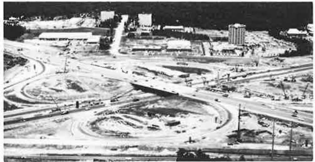
Figure 2. I-85 and I-285 interchange in northeast Atlanta: ramps relocated to allow construction of supports for new interchange ramps. (Hallman photo)
