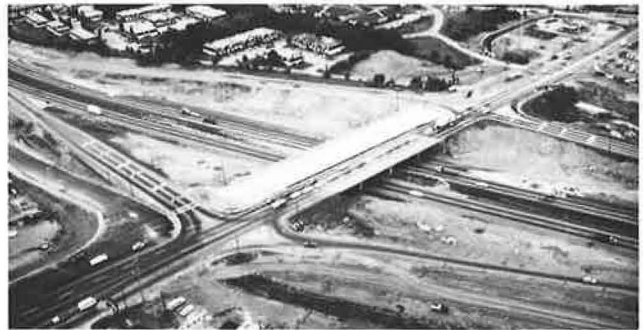
Figure 3. I-285 and Riverdale Road interchange: widening while maintaining traffic flow. (Hallman photo)
