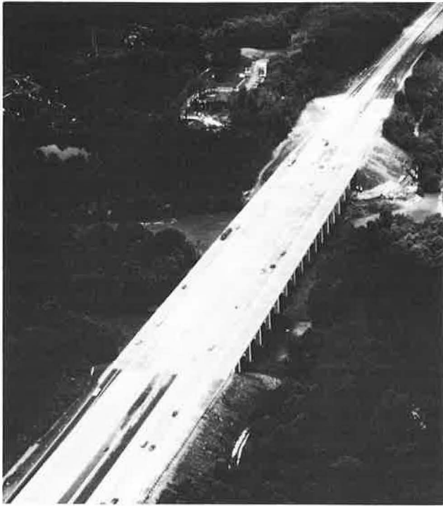
Figure 1. I-75 at the Chattahoochee River: bridge widening while maintaining two lanes of traffic in each direction. (Photo by Randy Hallman)
