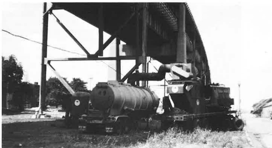
Sandblasting dust and debris are exhausted from enclosure above the disposal truck ( left ) and through water scrubber ( right ) to purify air.
