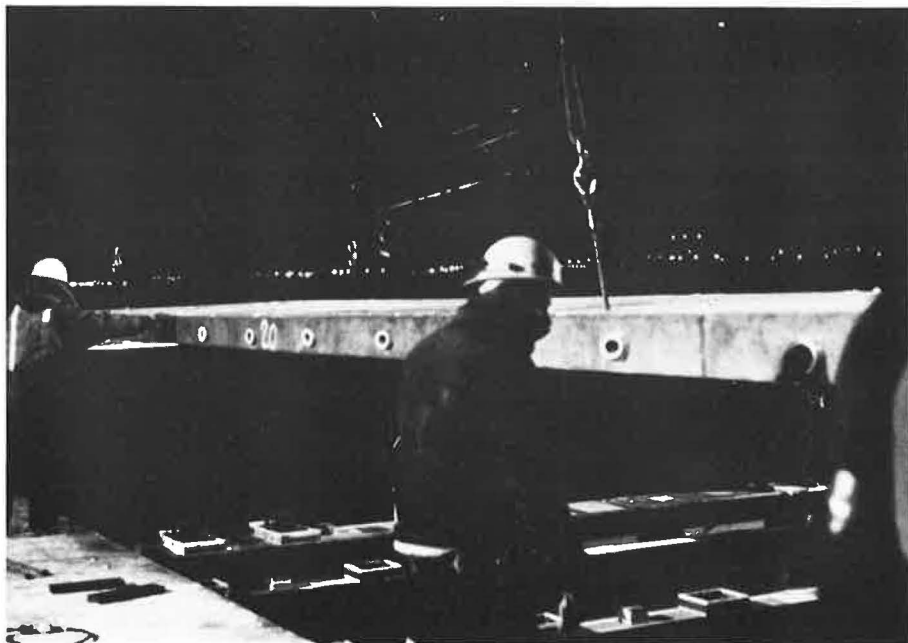
Precast deck panel is lowered into place during nighttime construction work. Ovals are ducts for longitudinal post-tensioning.
