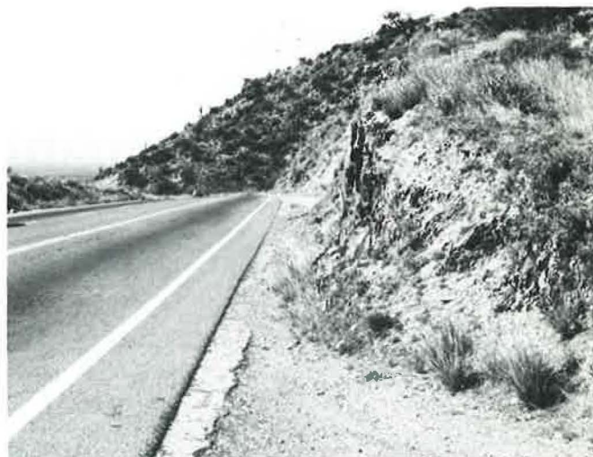
Widening lanes and shoulders in mountainous terrain is often costly, particularly where rock cutting is involved.
