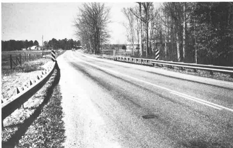
A secondary system RRR project that included lane widening, addition of a shoulder, and new bridge-approach treatment.
