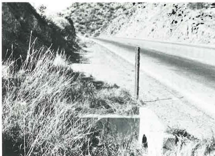
Culvert headwalls are a common roadside hazard. The problem has been mitigated in some RRR projects by extending the culverts, installing guardrails, or using special delineation treatments.
