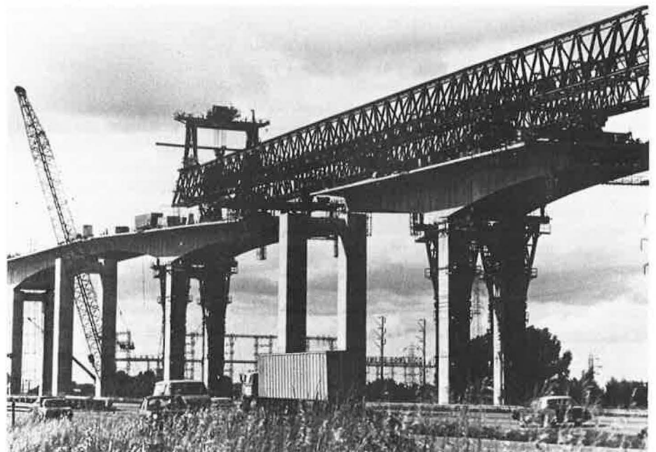
Figure 3. Deflected cantilever in Zilwaukee Bridge, Saginaw, Michigan. (photograph courtesy of Michigan Department of Transportation)
