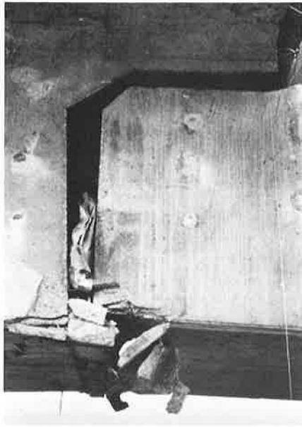
Figure 4. Spalled compressive region of "blocked" joint in Zilwaukee Bridge. (photograph courtesy of Michigan Department of Transportation)
