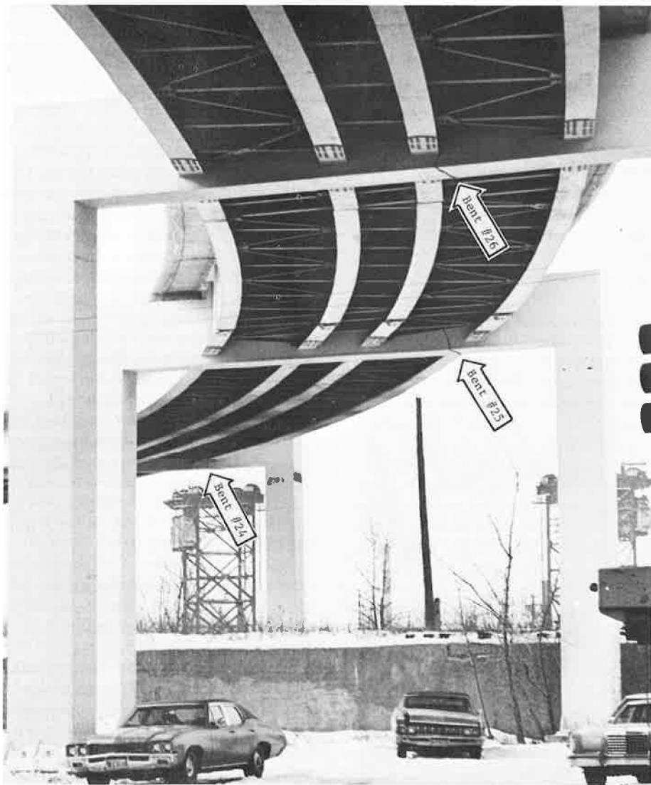
Figure 1. Cracked bents in Dan Ryan Rapid Transit, Chicago (arrows point to location of fractures). (photograph courtesy of Chicago Department of Public Works)
