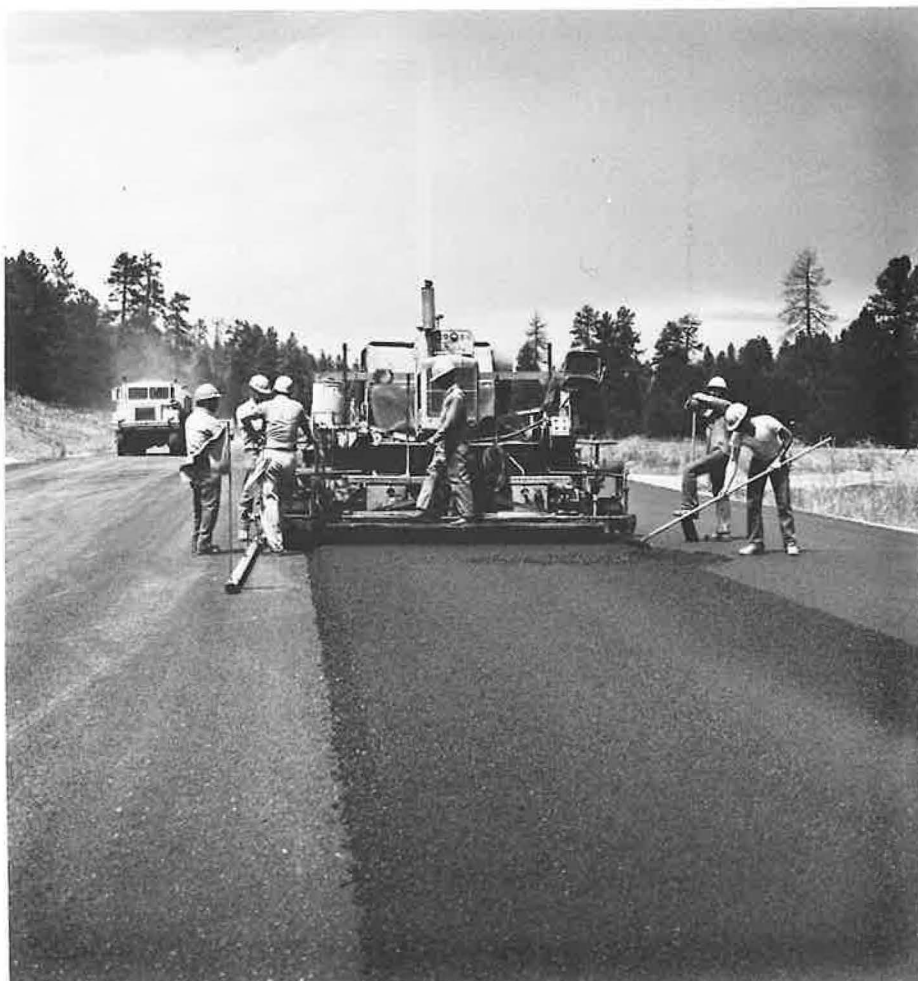
Asphalt concrete paving operations.
