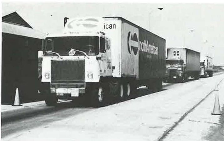
More energy-efficient vehicles and operations continue to be developed for all modes of transportation. This truck design incorporates a windshield to diminish air resistance.
