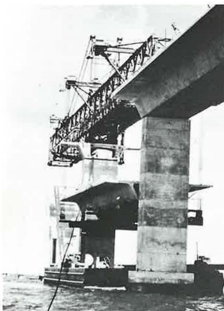
Seven Mile Bridge under construction in the Florida Keys. Completed in 1932, it is currently the longest continuous segmental bridge in the world: 35,000 ft.
