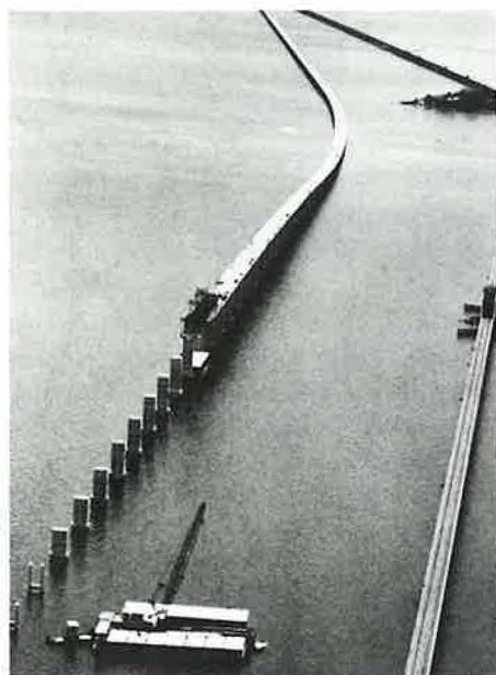
Seven Mile Bridge under construction in the Florida Keys. Completed in 1932, it is currently the longest continuous segmental bridge in the world: 35,000 ft.
