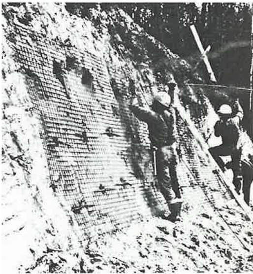
below FIGURE 14 Soil nailing for improving cut slope stability.
