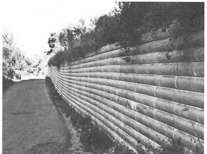
FIGURE 3 First highway use of modern earth reinforced wall: in France between Nice and the Italian border.
