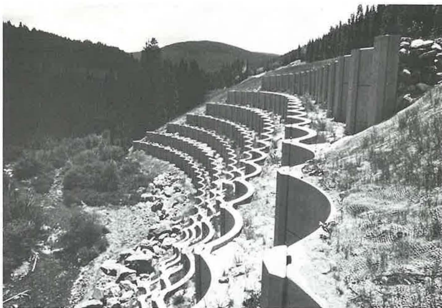
FIGURE 7 Special facing panels for reinforced earth wall along Interstate Highway 70 through Vail Pass, Colorado.
