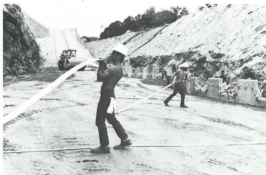
FIGURE 18 Reinforcement placement.
