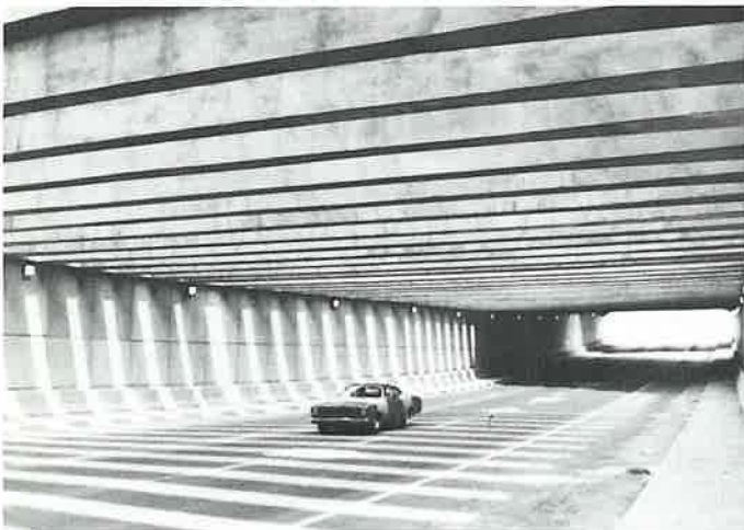
FIGURE 12 Strutted, slurry wall carrying depressed I-75 ramp, Atlanta.
