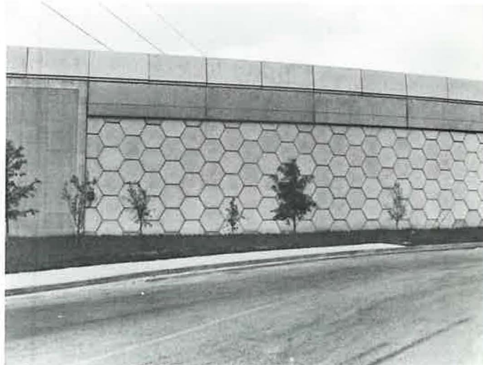
FIGURE 5 VSL wall supporting MARTA rail line over Piedmont Avenue, Atlanta.
