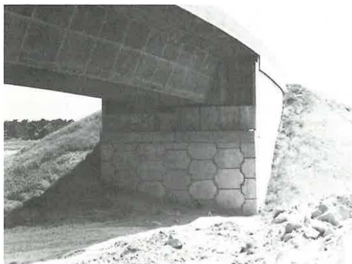
FIGURE 9 GASE wall abutment at I-85/I-285 interchange Southwest, Atlanta.
