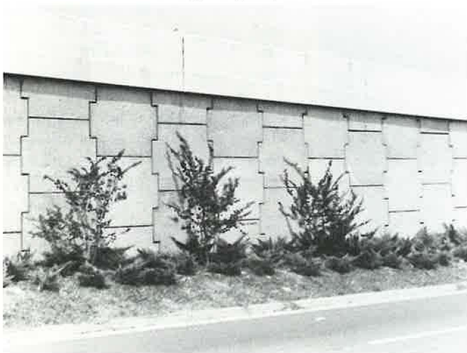
FIGURE 2 RE wall detail supporting I-85, Atlanta.
