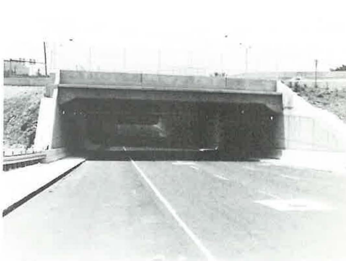
FIGURE 11 Strutted, slurry wall, I-75, Atlanta.
