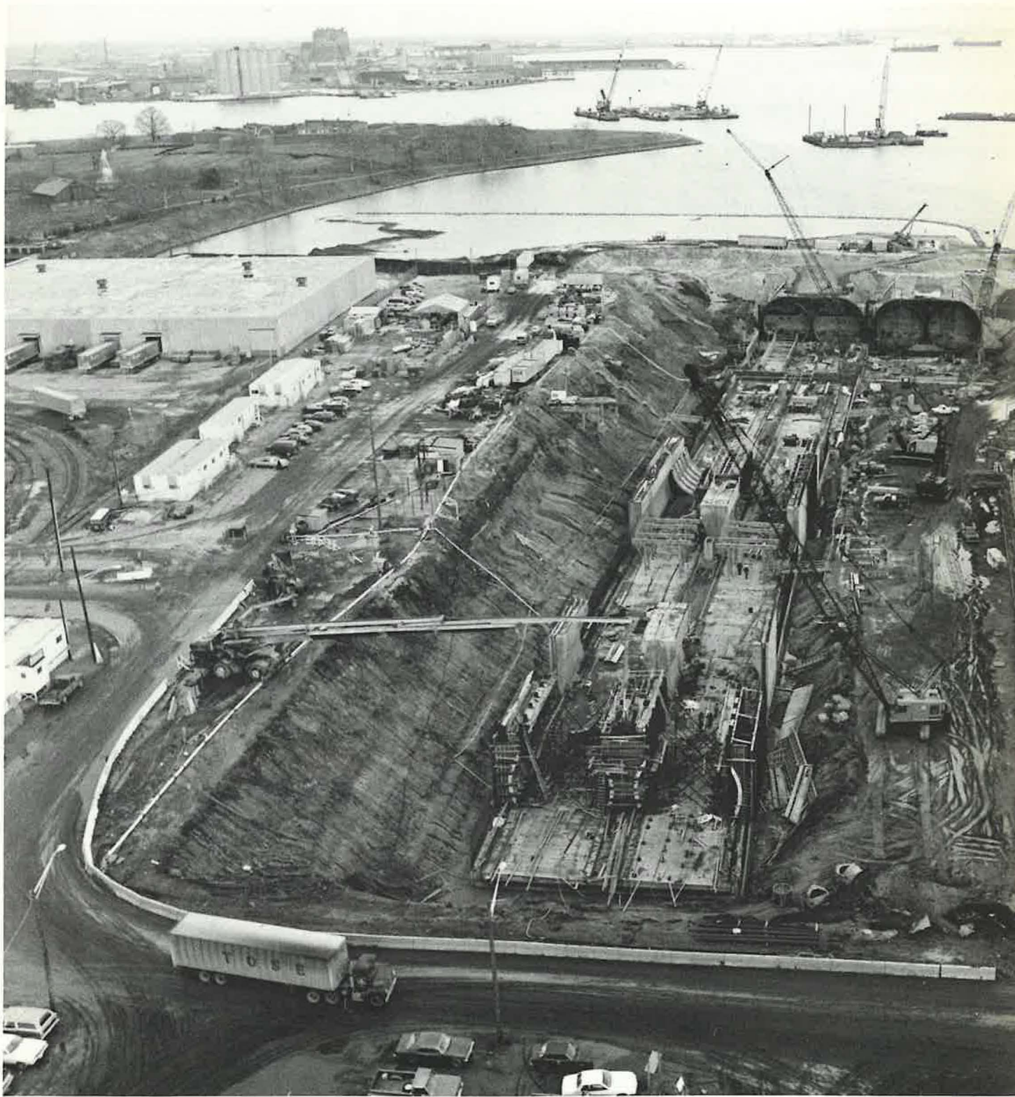
West portal of the Fort McHenry Tunnel during construction. Extensive dewatering of the excavation was necessary. Note the submerged tube modules at far end of excavation.
