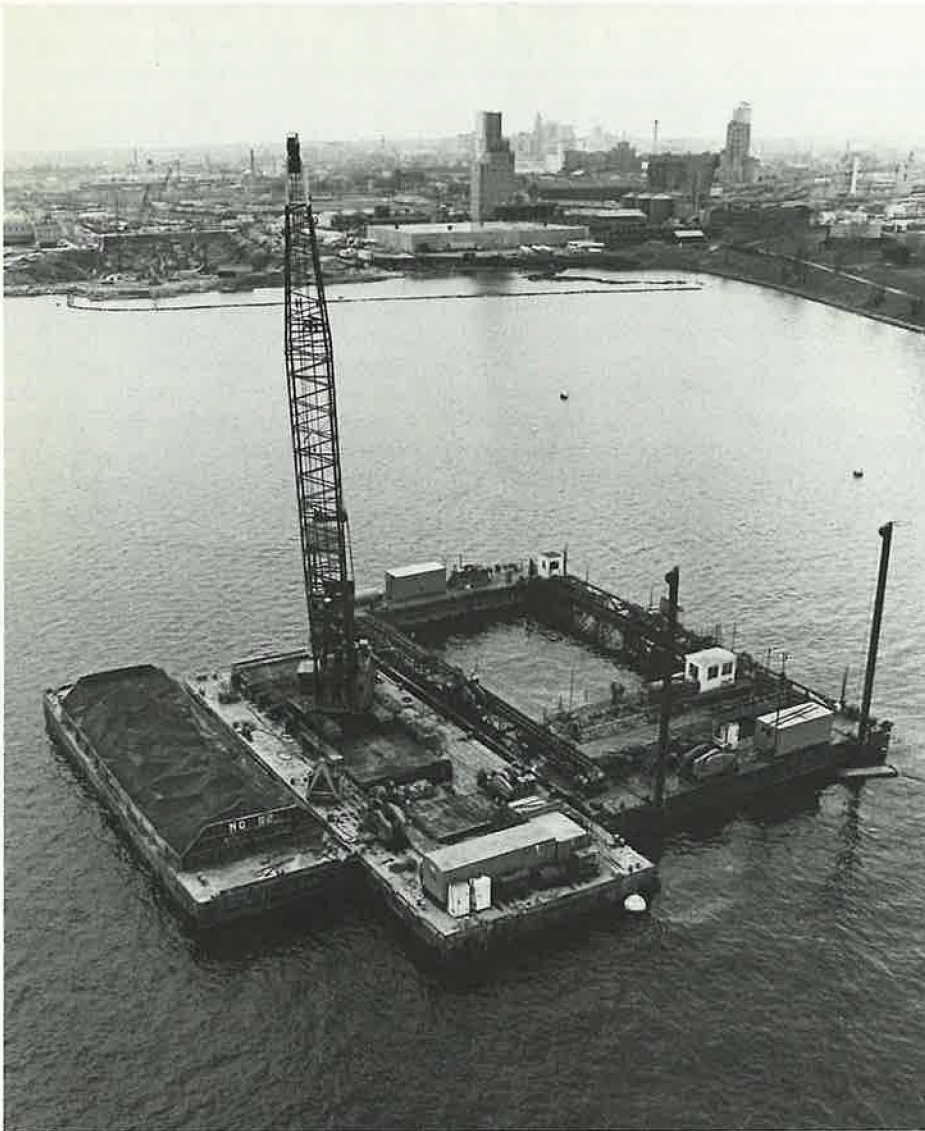
Gravel barge and floating screed during construction process. Procedures for preparation of the gravel bed in the dredged harbor floor trench were critical; improper grade control would have prevented proper placement of tube modules.
