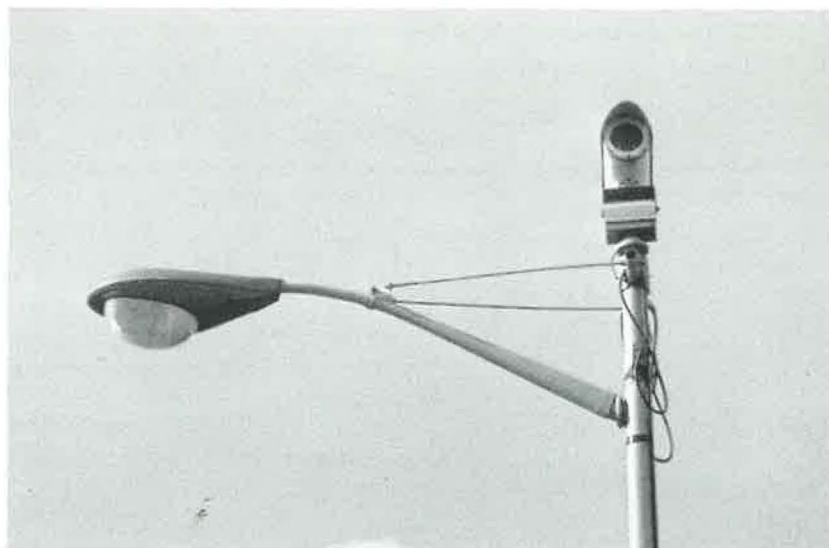
Surveillance camera for monitoring freeway conditions.
