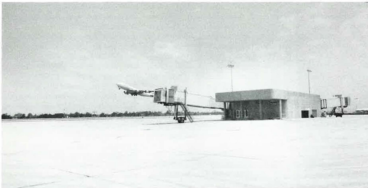
FIGURE 8 Remote satellite passenger boarding facility, designed for the Los Angeles International Airport, is capable of accommodating all sizes of aircraft. The facility includes four loading bridges, concourses to the ground level, and bus parking facilities to transport passengers to and from the terminal.
