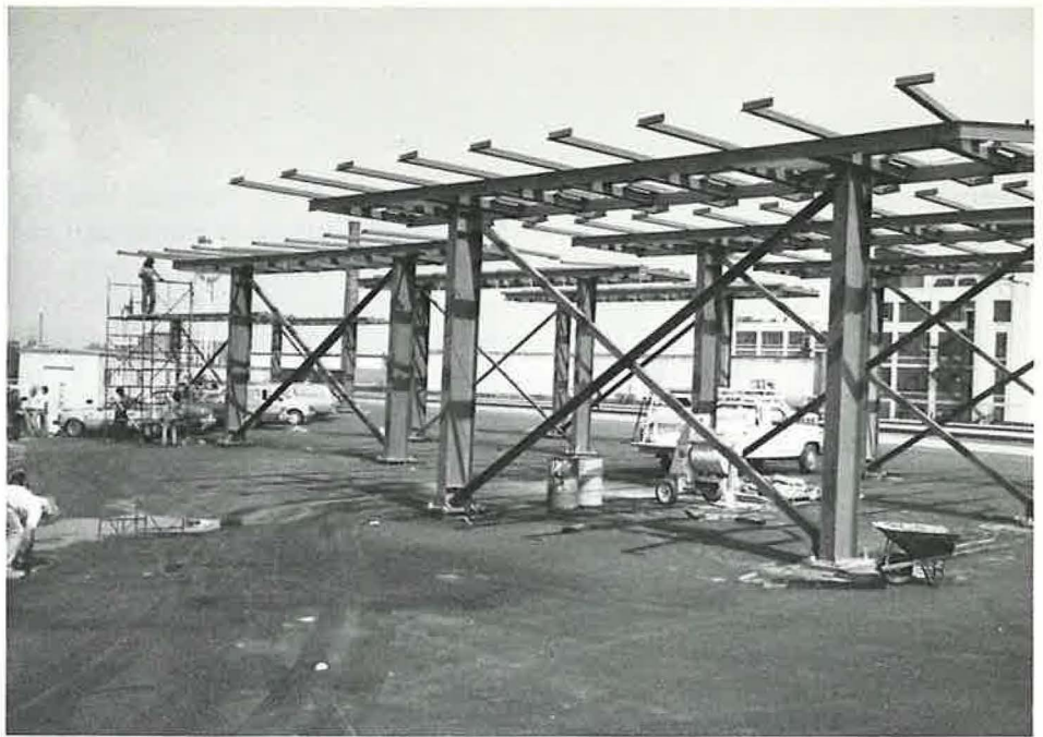
Trailer chassis-stacker facility. At Global One empty trailers will be stacked vertically to save storage space. They are lifted into the stacker via forklift.
