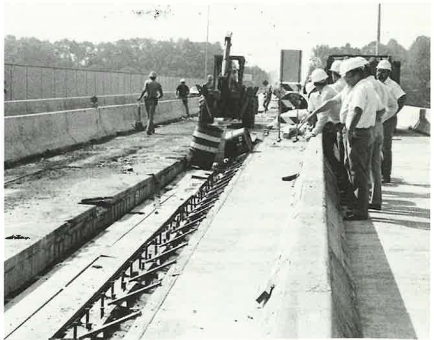
Members of the TRB Committee on Structures Maintenance observe the process of replacing and widening a deteriorated bridge deck.
