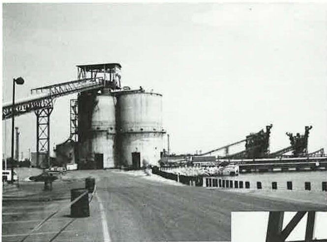
Coal transfer facilities at the Dominion Terminal. Coal is picked up from ground storage areas, blended in the twin silos, and loaded on shipboard at the rate of 6,500 tons per hour.
