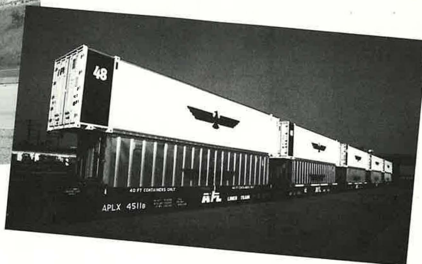
Changing relationships between ocean carriers and railroads have been enhanced by the rapid growth in double-stack trains, allowing for the efficient and cost-effective movement of containers to inland destinations. (photograph from American President Companies, Ltd.)
