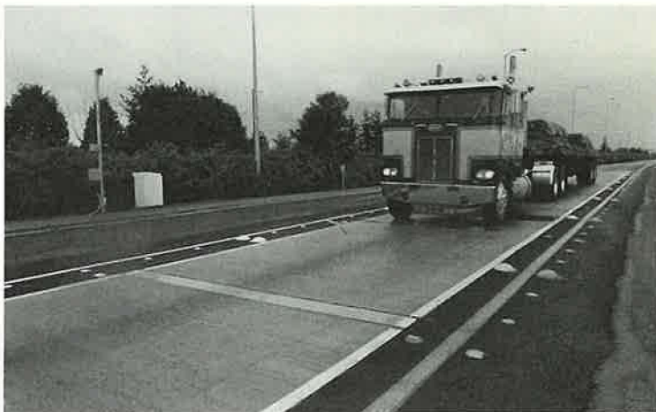
Truck approaches slow-speed weigh-in-motion and automatic vehicle identification site at Woodburn, Oregon, weigh station.
