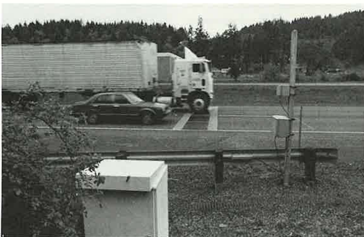
One of Oregon's 350 transponder-equipped heavy vehicles crossing a fast-speed weigh-in-motion and automatic vehicle classification station. Data collected for planning purposes include time, vehicle weight, and speed.
