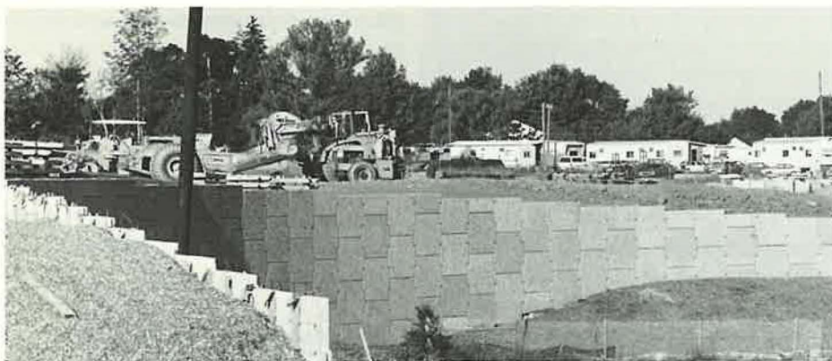
Use of engineering fabrics and soil reinforcement is becoming more common for the construction of embankments and retaining walls.
