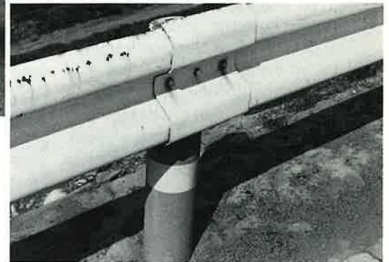
Closeup view of guardrail installation.
