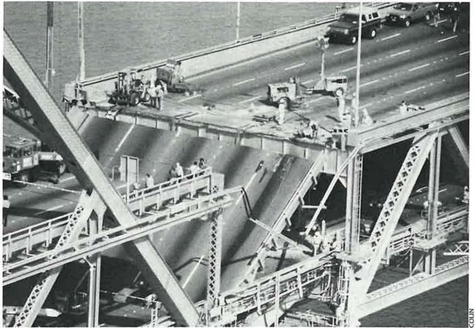
San Francisco-Oakland Bay Bridge failure after anchor bolts on truss span gave way, resulting in collapse of two closure deck spans.
