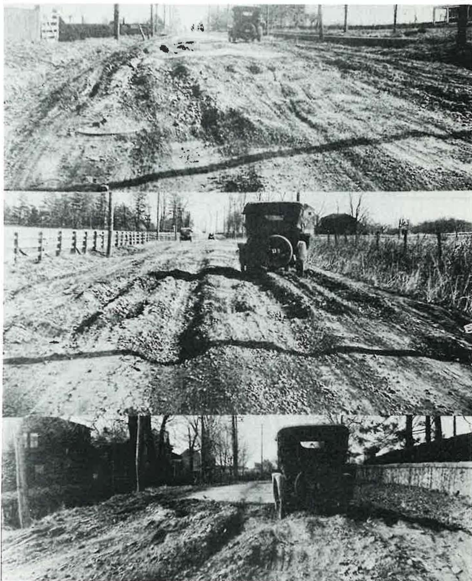
Damage to Philadelphia Pike in Wilmington, Delaware, after passage of fleet of 100 heavy trucks.
