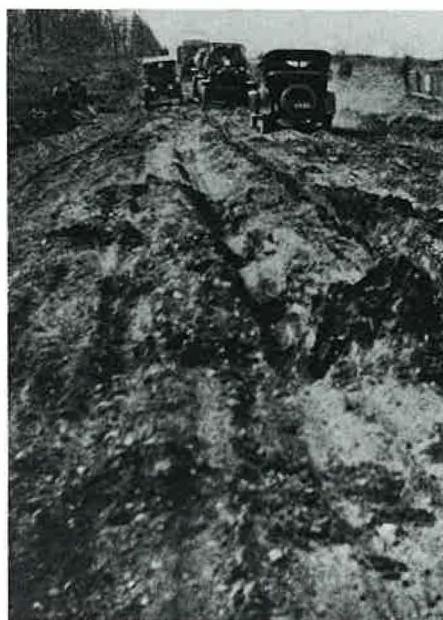
Section of road near Canandaigua, New York, destroyed by seven-ton trucks during World War I.
