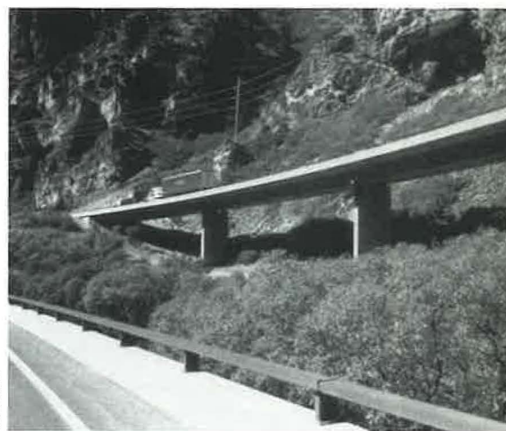
Pier shapes and bridge rail are two components specifically developed for and standardized throughout the project.
