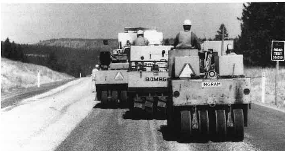
SPS-3 site on US-195 near Spokane, Washington, where the effectiveness of four preventive maintenance treatments will be tested, including chip seal overlays, shown here under construction.
