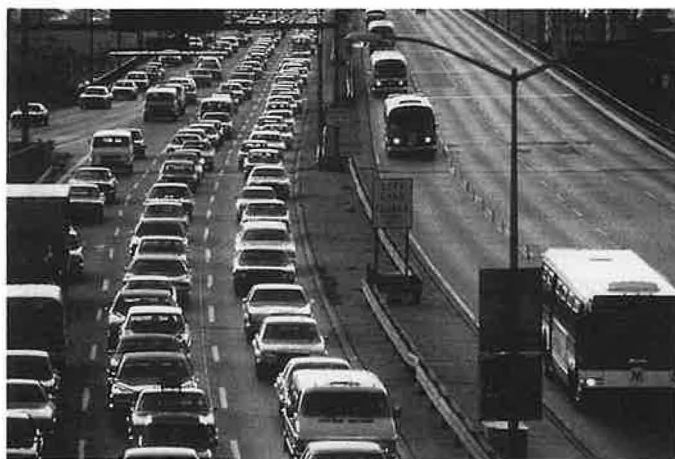
FIGURE 3 Examples of HOV facilities: (a) exclusive HOV facility in freeway right-of-way: I-10 West (Katy) HOV lane, Houston, Texas, (b) concurrent flow lane: SR 520 HOV lane, Seattle, Washington, and (c) contraflow lane: Gowanus Expressway HOV lane, New York City.
