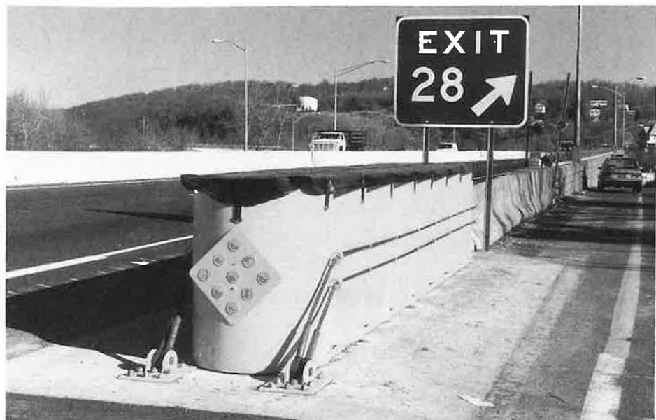
Narrow Connecticut Impact Attenuation System developed by ConnDOT has been successfully crash tested and approved for use on Federal-aid highways.
