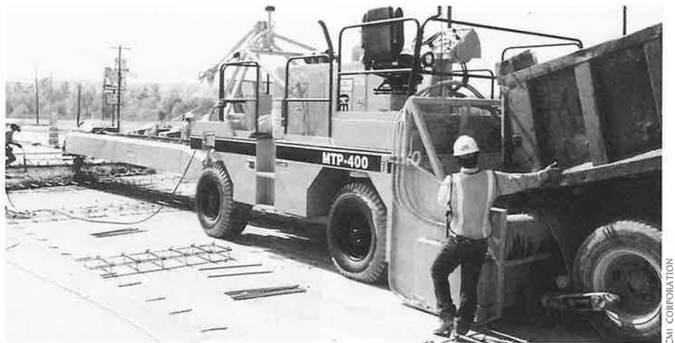
Concrete material transfer/placer. Quality in construction is receiving renewed national emphasis.
