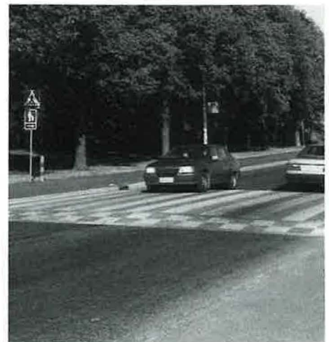
Pedestrian crosswalk on popular scenic road in Helsinki, Finland, doubles as traffic-calming speed hump.
