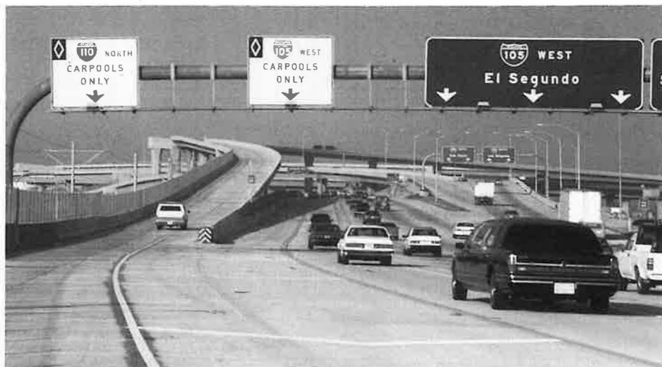
To connect one HOV lane to another, ramps are being constructed in freeway interchanges (ramp between I-105 and I-110 in Los Angeles).
