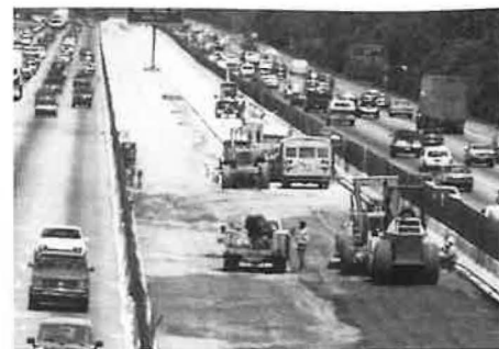
Most HOV lanes are being added by modest widening and freeway construction (I-405 in Orange County, California).
